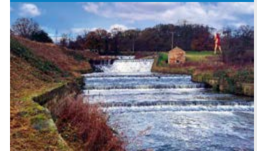
RESERVOIR SAFETY & REPAIR
