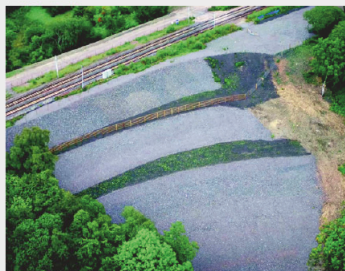
Geotechnical and earthworks
