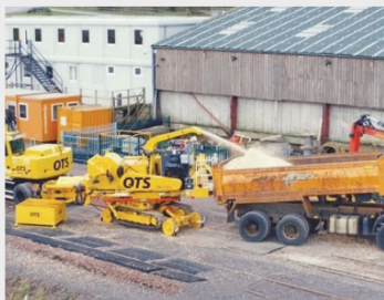
Civil asset management
